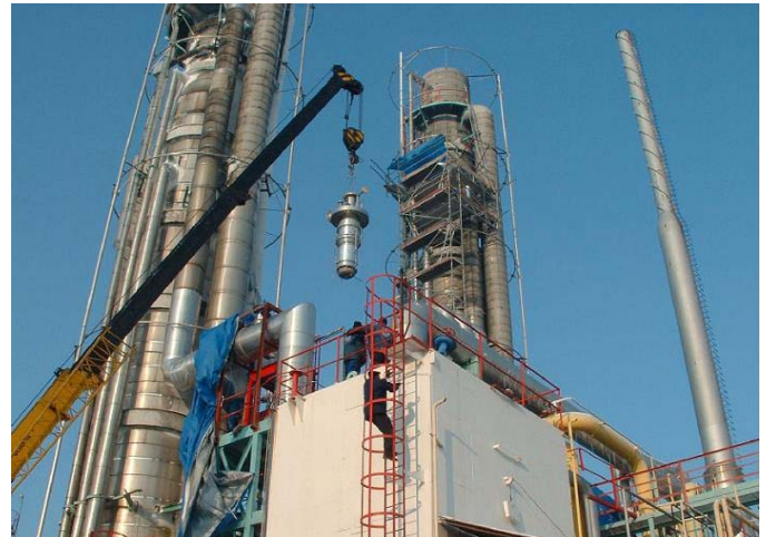
Figure 17: Installation of the Very First Two-Phase LNG Expander in Poland 2003
