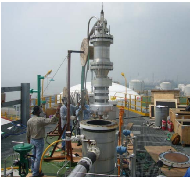
Figure 1: Installation of EIC In-Tank Ammonia Pump
