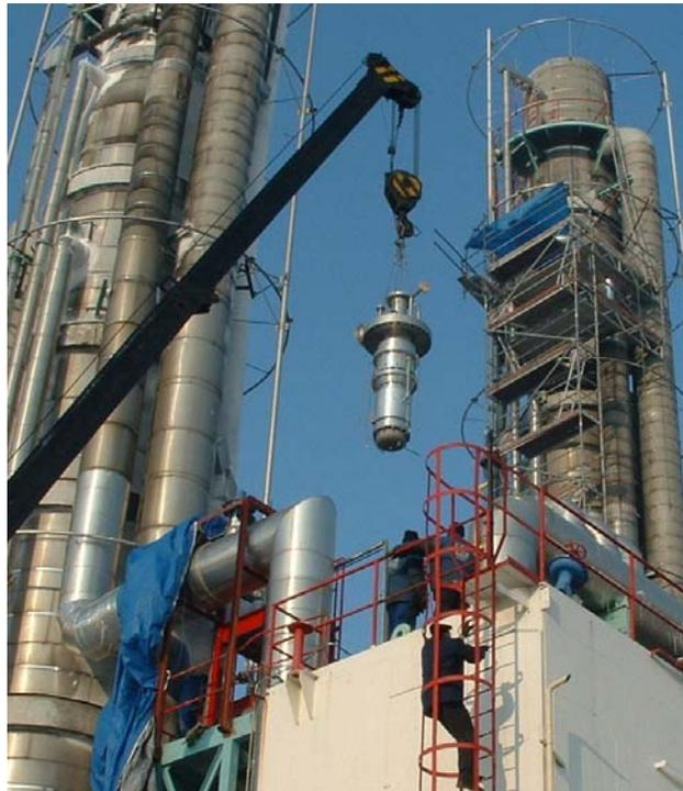
Fig. 3: Installation of EIC two-phase expander
